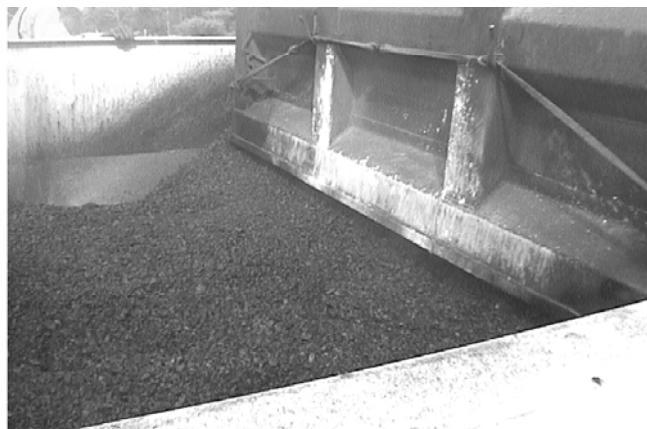
Flooding hopper with HMA
