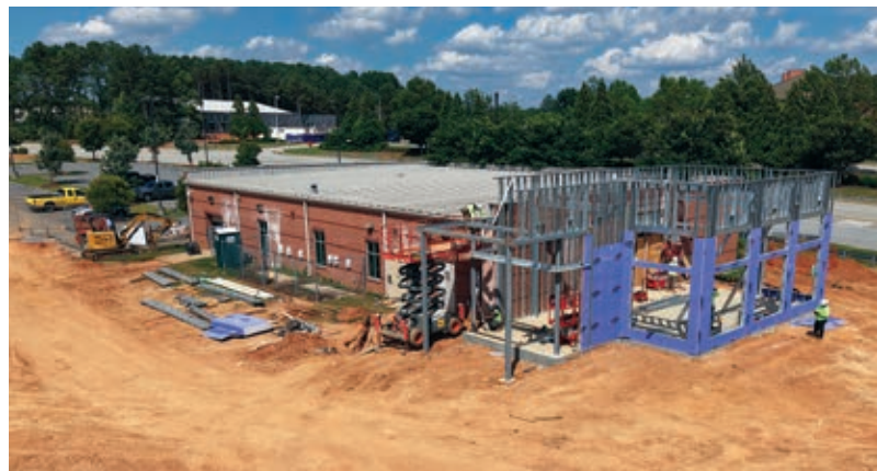
A new lobby is being added to the Corporate and Community Education building at the Anderson Campus.
