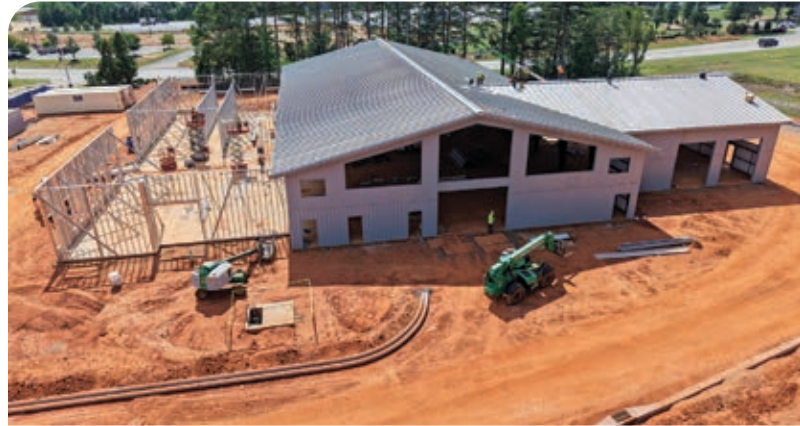
Classroom and office framing for the Automotive and Diesel Labs at the Anderson Campus.
