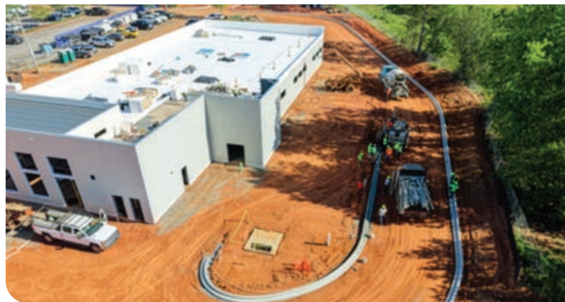
Curbing and gutters on the Mechatronics building at the Anderson Campus.
